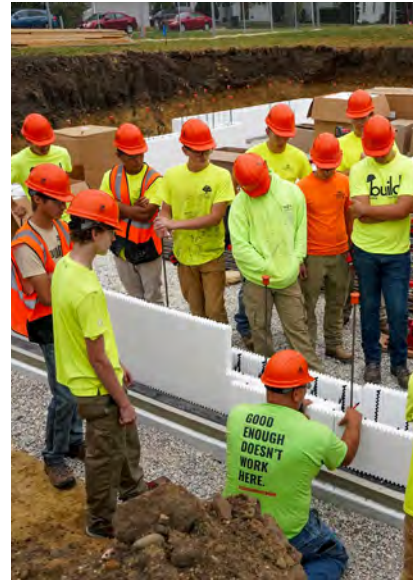
First-year students in the Sustainable Construction and Design program at Hawkeye Community College in Waterloo, Iowa, learn about building a foundation. Photo courtesy of Hawkeye Community College.
